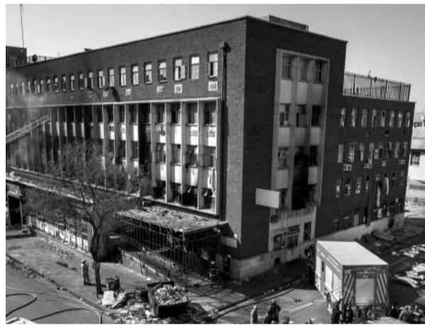
ict downtown apartment building that was inhabited by mainly homeless people and others who
